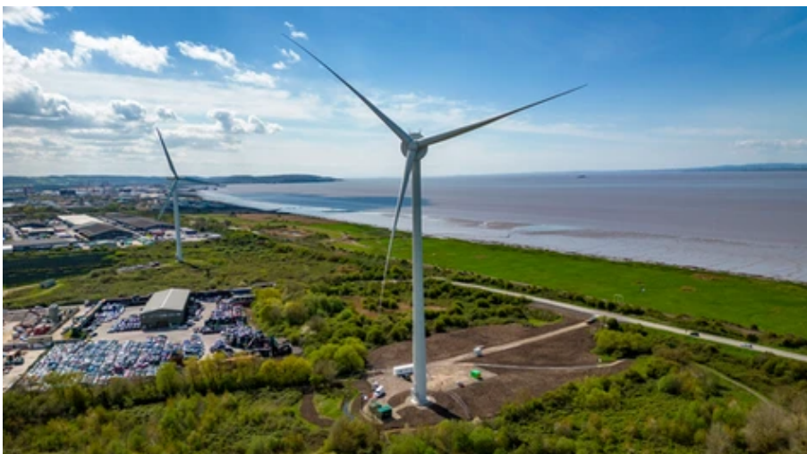
Photo: Ambition Lawrence Weston turbine in operation 15
