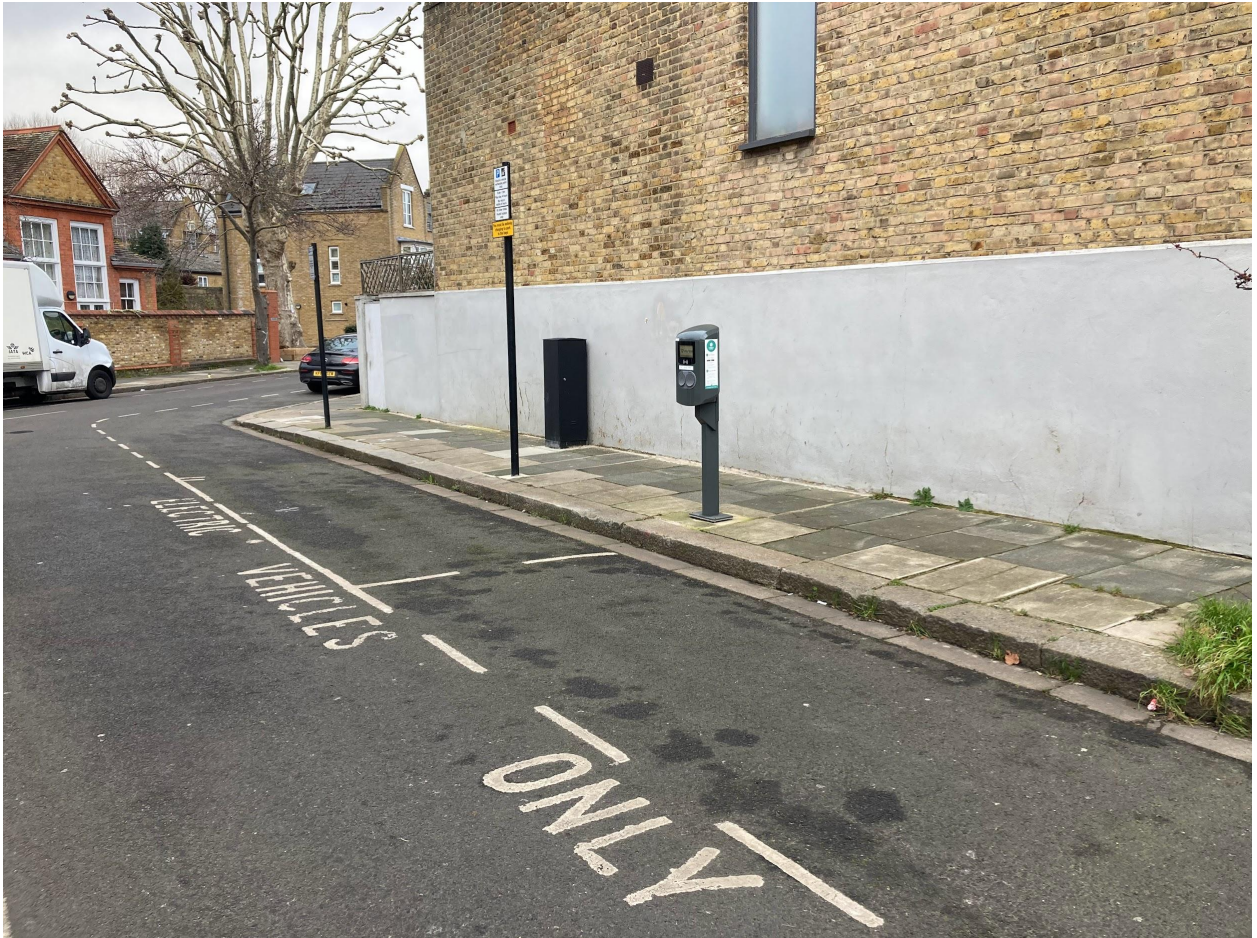
Figure 15: Vespan Road, Liberty Charge double chargepoint, typical arrangement. Credit: Possible.
