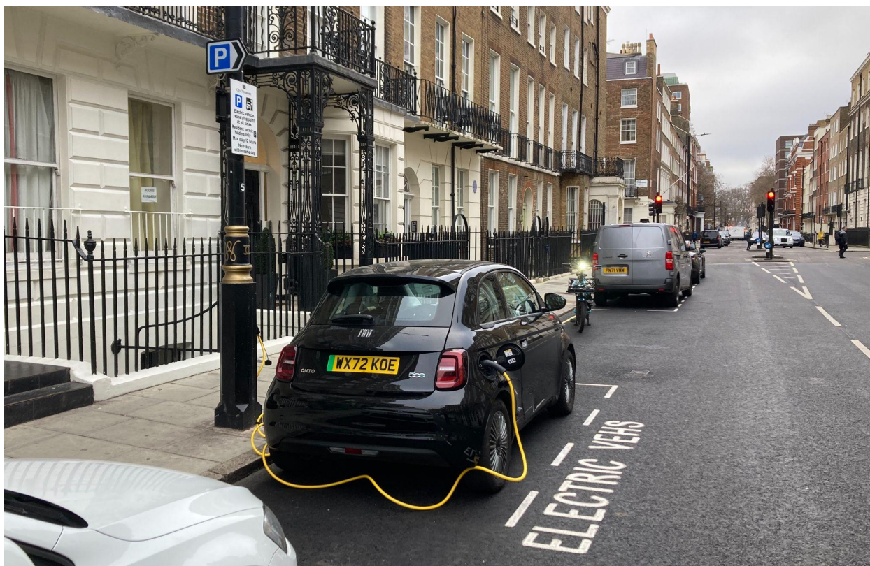
Figure 14: Example of a lamppost charger in use in Westminster. It is not accessible to Disabled drivers. Credit: Possible
