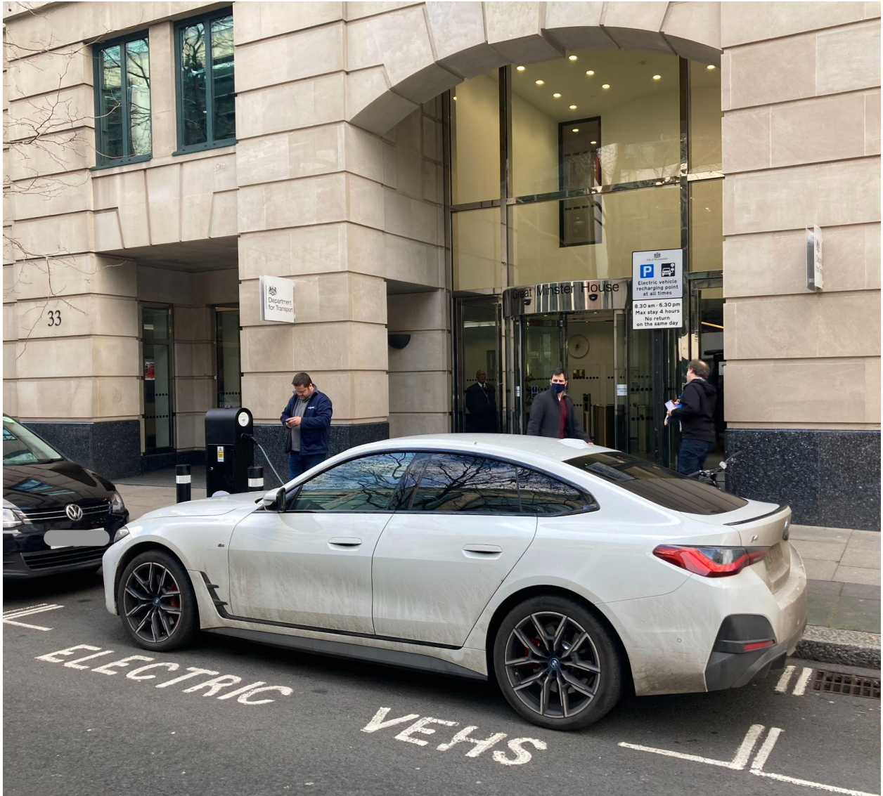
Figure 12: EV chargepoint installed by Westminster Council on the pavement directly outside the entrance to the Department for Transport, whose own best practice guidance specifies they should be sited in the carriageway. A kerb buildout could have been easily accommodated between parking spaces here.
