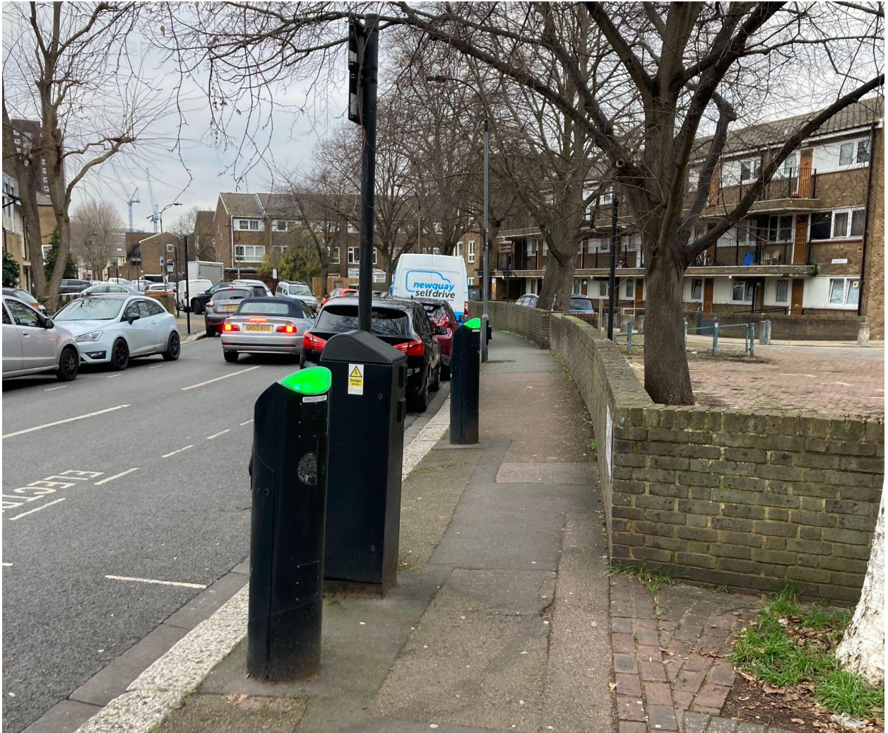
Figure 16: Everington Street, Source London chargepoints. These have not been made accessible for Disabled drivers. Credit: Possible.
